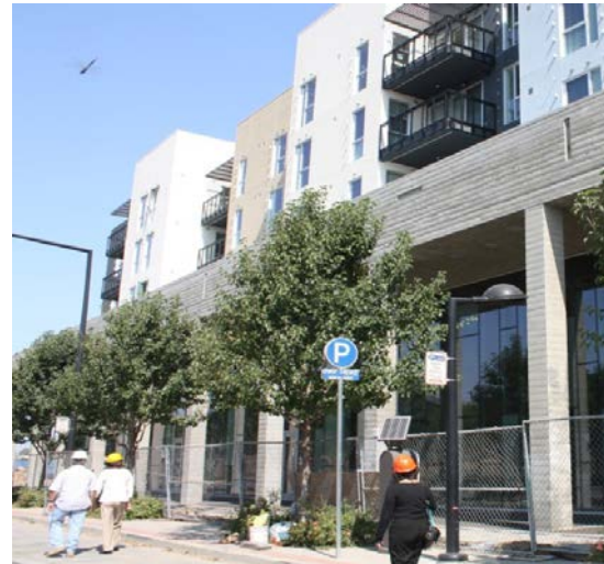
Union City Intermodal, Union City $8M TOD Grant 344 Total Units 155 Affordable
